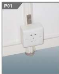
插座 Power Socket(Square Pin) Max.500W
